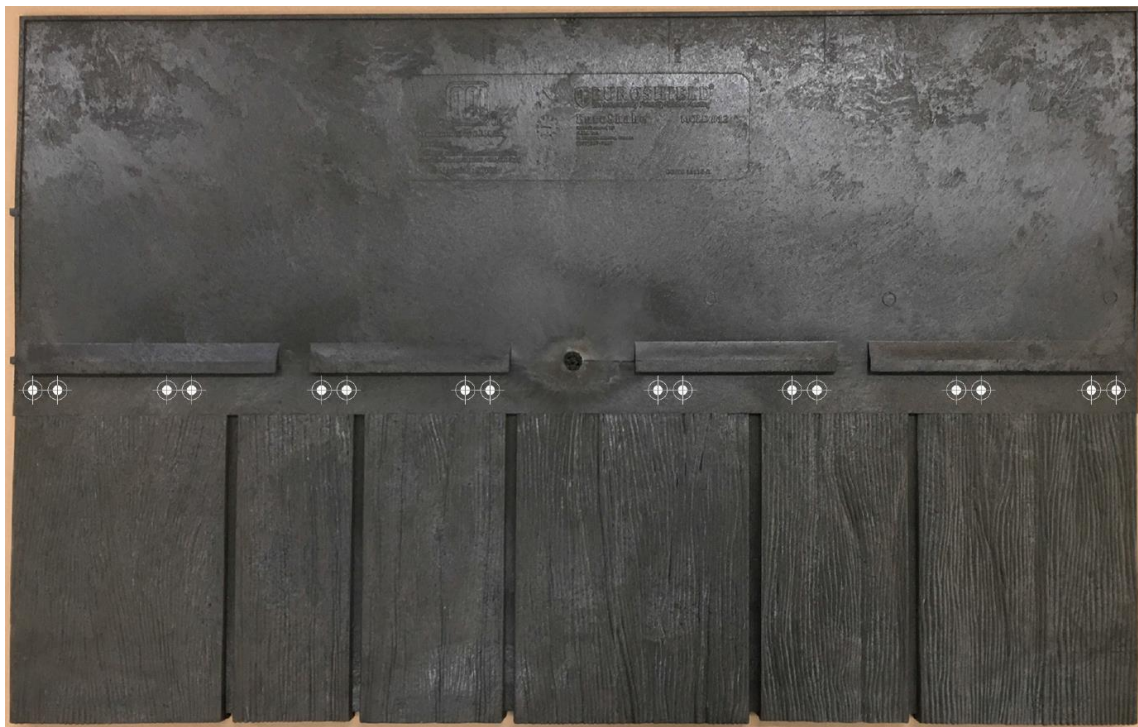
Figure 4: 16 nails/shingle installation of Ranchlands Shake
